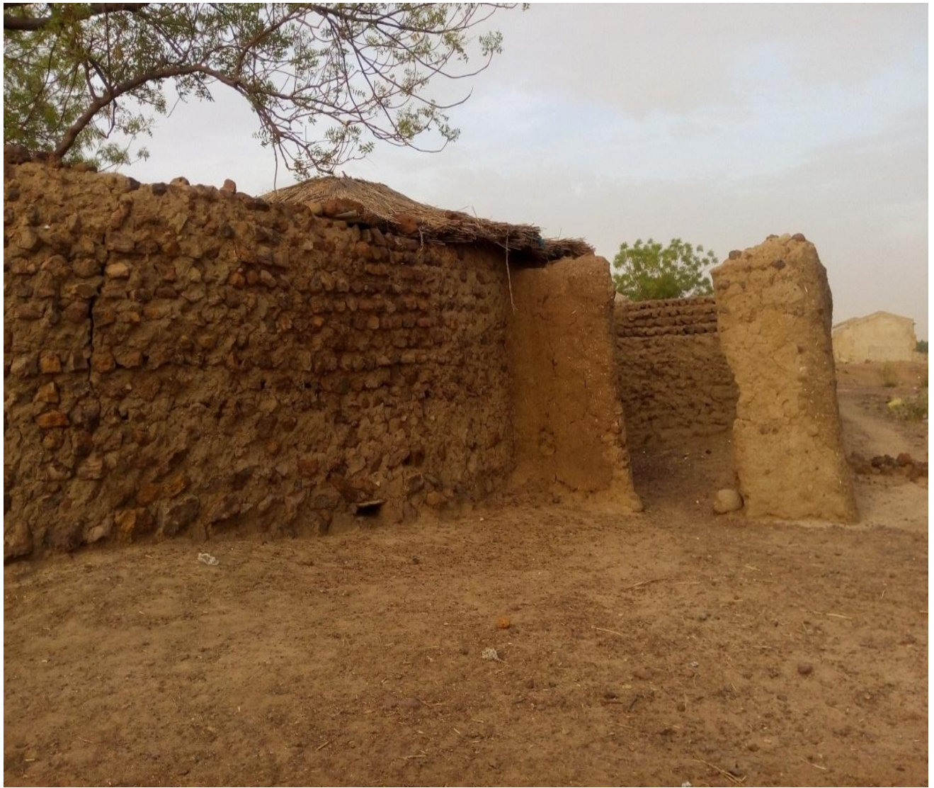
Figure 4.17a: Photograph of the Typical Mud Residential Building in Rimawa Flood-Affected Area
